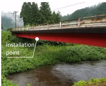
Target bridge and Installation location.
